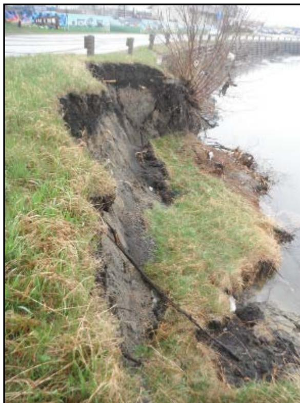
**Figure 3: Stream Bank Failure on the Sheyenne River**
